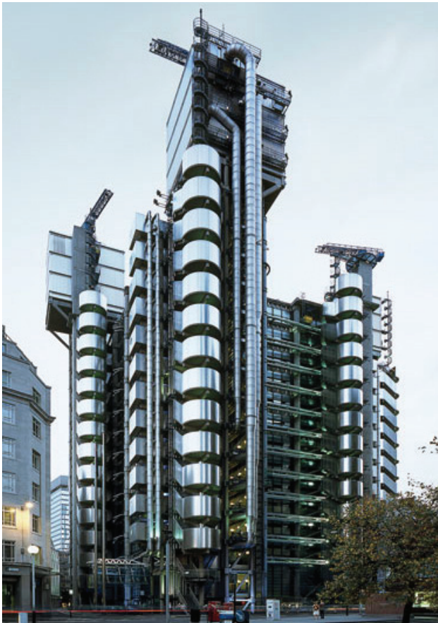
Richard Rogers, Lloyd's building London
